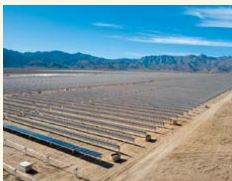
Mexico: Solar power generation facilities (Photo: IEnova)
