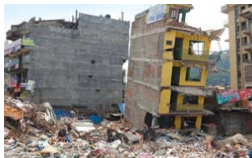
Nepal: Collapsed buildings in the April 2015 earthquake
